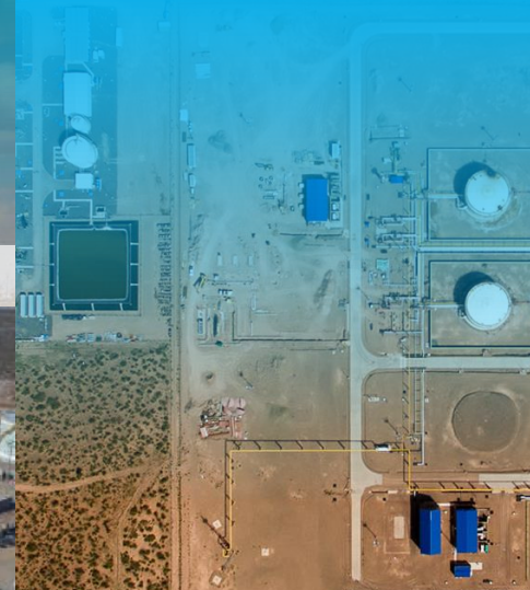
BANDURRIA SUR OIL TREATMENT FACILITY
