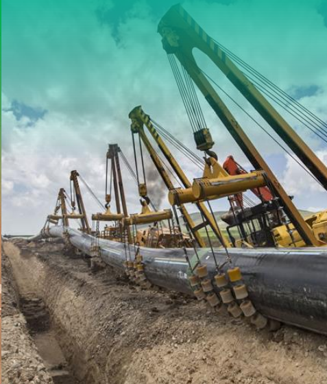
LC-PELLEGRINI OIL PIPELINE
